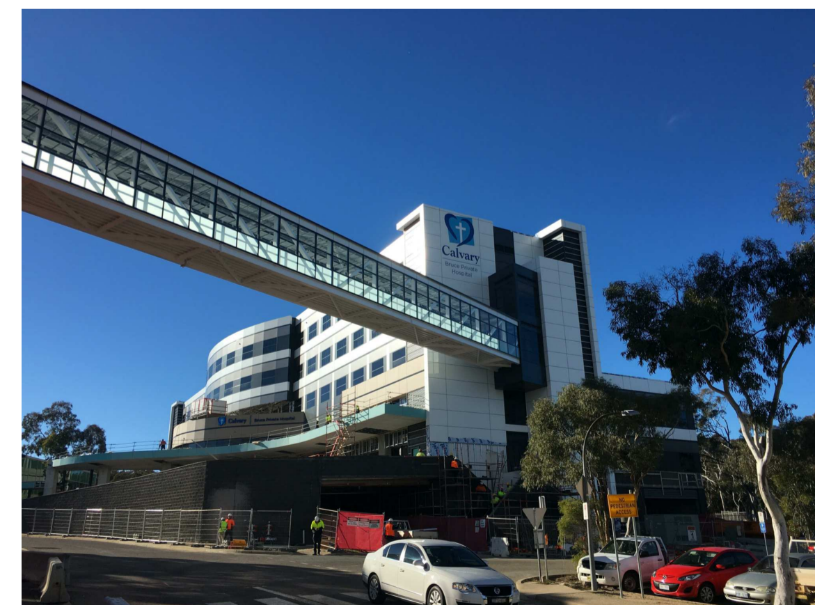
EXAMPLE OF VISIBLE STRUCTURAL COLUMNS
