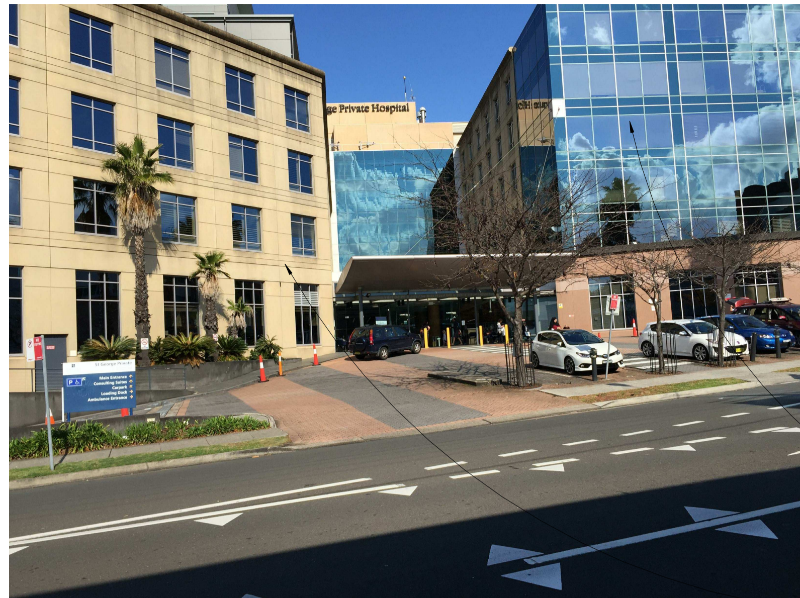
EXTERIOR VIEW OF EXISTING ST GEORGE PRIVATE HOSPITAL
